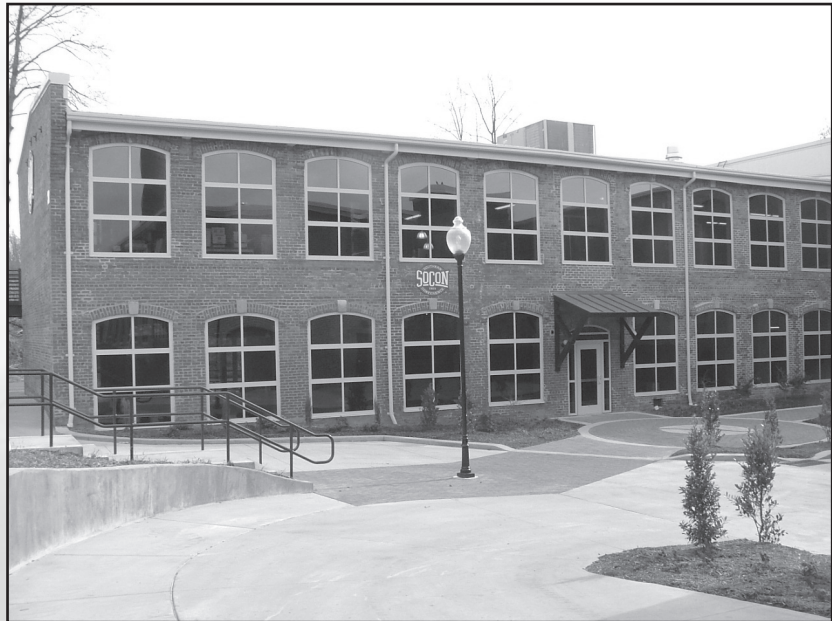
The Southern Conference moved its offices into the historic Beaumont Mill in Spartanburg, SC in January, 2005. The mill was constructed in 1890 alongside Chinquapin Creek. The main products in 1900 were carpet warps, seamless bags (for corn and grain), and wrapping twines for domestic market. In 1907, the mill operated with 12,360 spindles and 252 automatic looms. During WWII, Beaumont Mill produced "duck" which was the fabric made to outfit GIs in rafts and ammunition belts. The mill closed in 1999 and was partially dismantled in 2002. The Southern Conference was the first tenant in the revitalized mill.
